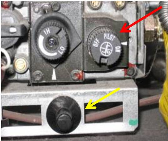
Turn the control knob (red arrow) so that the "Pilot" designation lines up with the white triangle.
