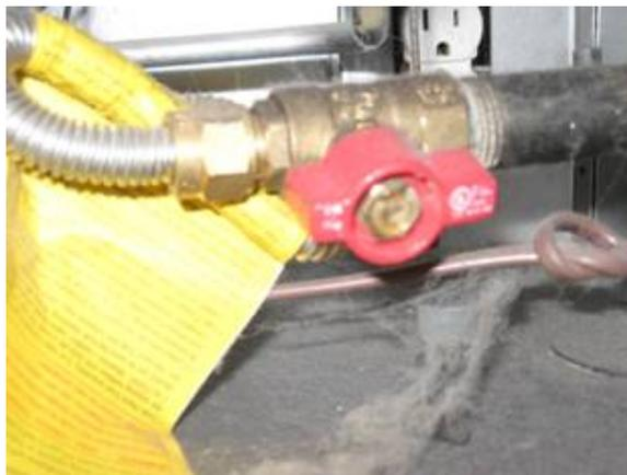
The red, yellow or blue gas line shut-off handle should be in the open position. The picture above shows the open position, parallel with the gas pipe. If the red handle were rotated 90 degrees, the valve would be in the off position, perpendicular to the pipe.
