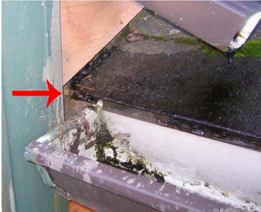
Here are some other telltale signs that kick-out flashing is either missing or improperly installed. Note the stains on the siding.
