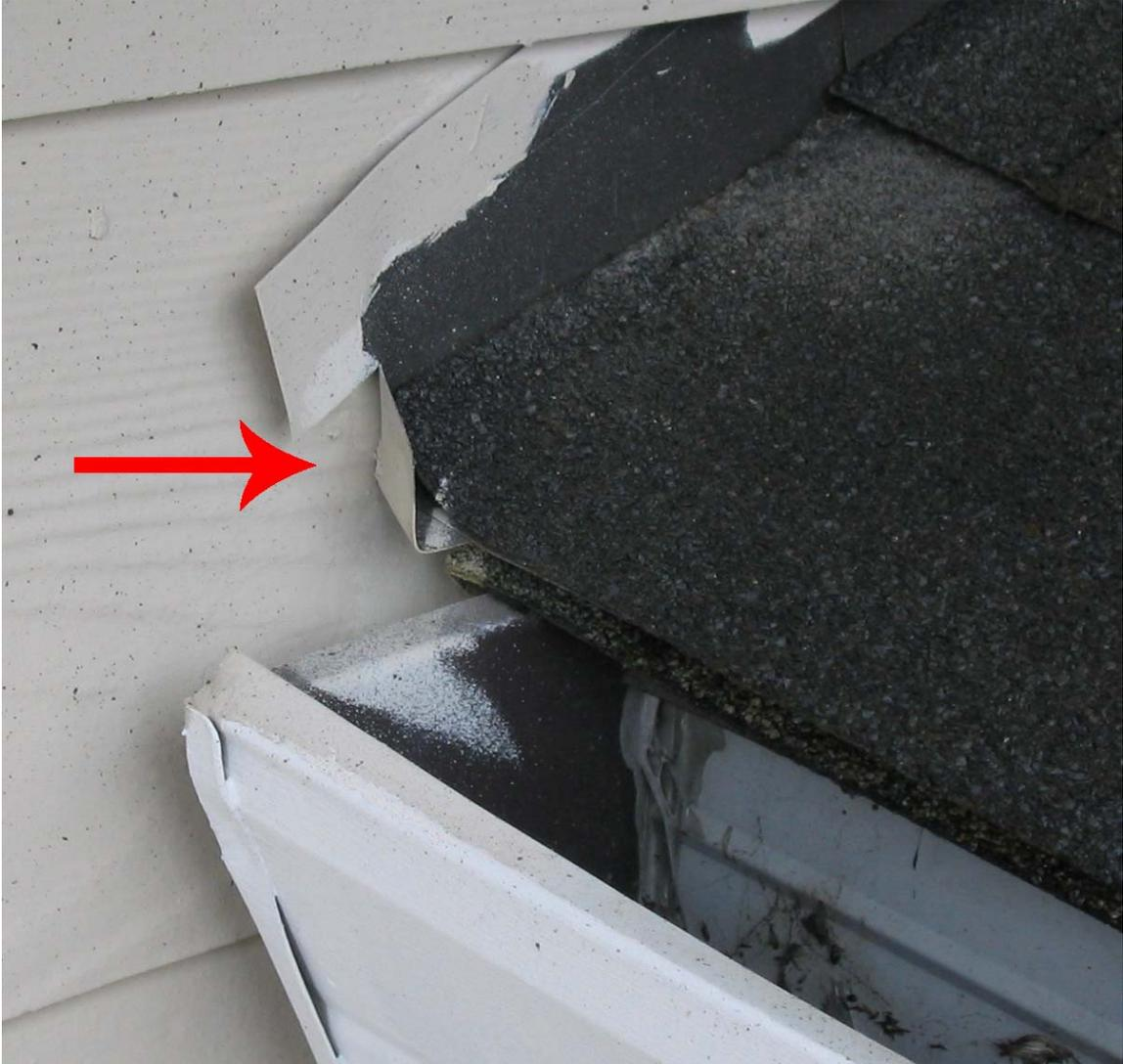
So now you can see the importance of a tiny piece of metal – it IS the little things that matter. Don't overlook gutter and downspout maintenance. It's extremely important for keeping your basement or crawlspace dry, and if you have areas that would require kick-out flashing, your siding and interior walls could even be in danger!
