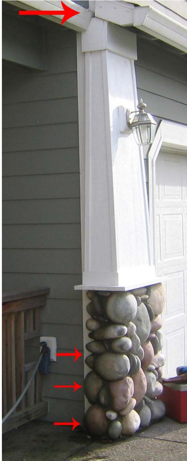
This photo shows an attempt to use proper diverter flashing but it is not extended far enough past the roof edge to allow water to get into the gutter:
