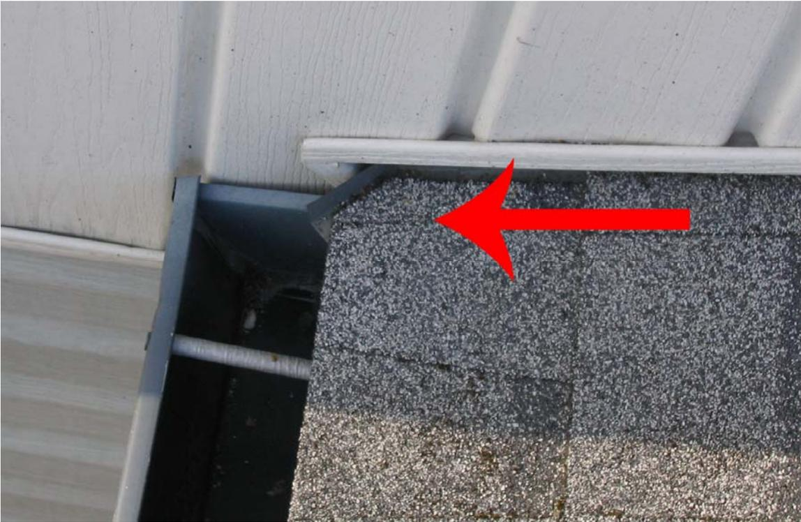
Here is a picture of inadequate kick-out flashing. Notice the gaps where water runs down the wall.
