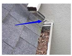
**45: -** The wall flashing is designed for a shake roof. The exposure is too much of a comp shingle. When the roof is replaced have the roofer replace all of the wall flashing to match the shingles being installed.
