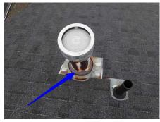
**61: -** In the attic, there are rust spots in the furnace vent and it's flashing. They don't appear to be leaking yet. Keep an eye on the and plan on replacing them when the furnace is replaced.
