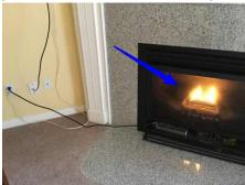
**67:** The heatolator fan has not been completely or properly installed. Hire a gas fireplace installer to finish installing this fan. The fan should be located in the back of this space under the firebox. The contractor should work with an electrician to get an outlet installed in the same space as the fan. The fan sounds fine otherwise:
