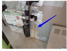
**165: -** In the jacket of the evaporator, the seals around the pipes are leaking air into the garage. This is a waste of energy. Have the heating contractor seal these openings.
